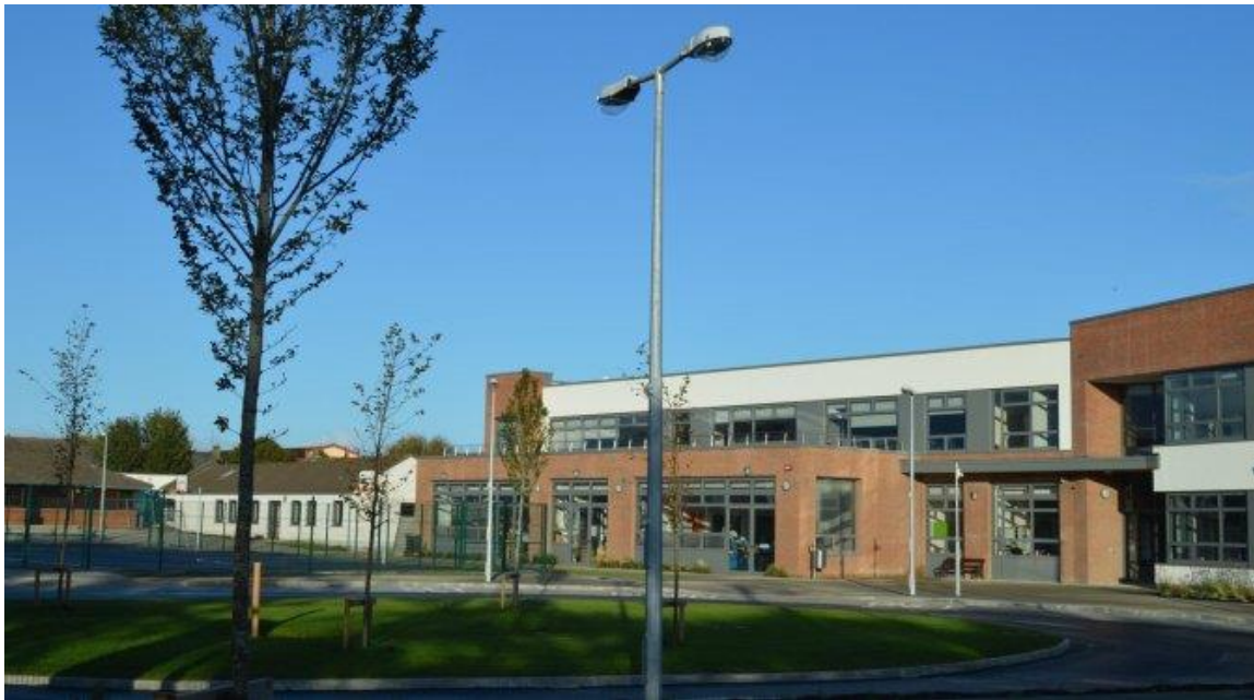
Completed extension at Coláiste Abbain
